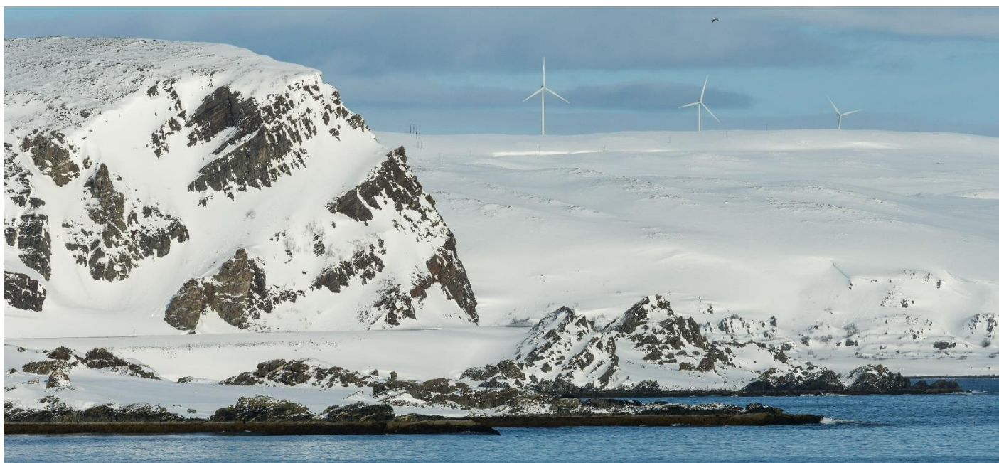
Figure 2 - Wind Power Plant Raggovidda (Norway)
