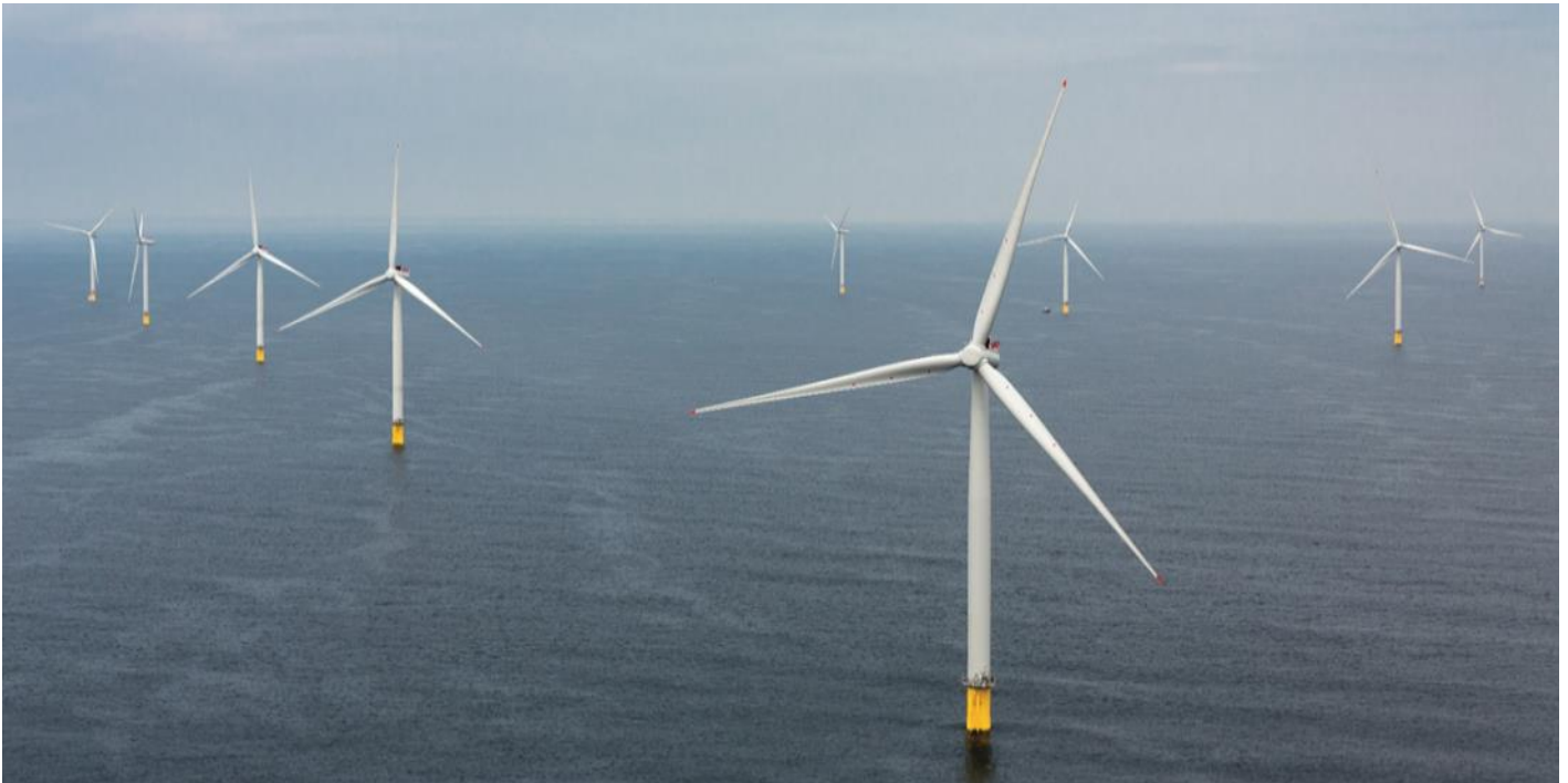
Figure 3 - Westermost Rough Offshore Wind Power Plant (North Sea, United Kingdom)
