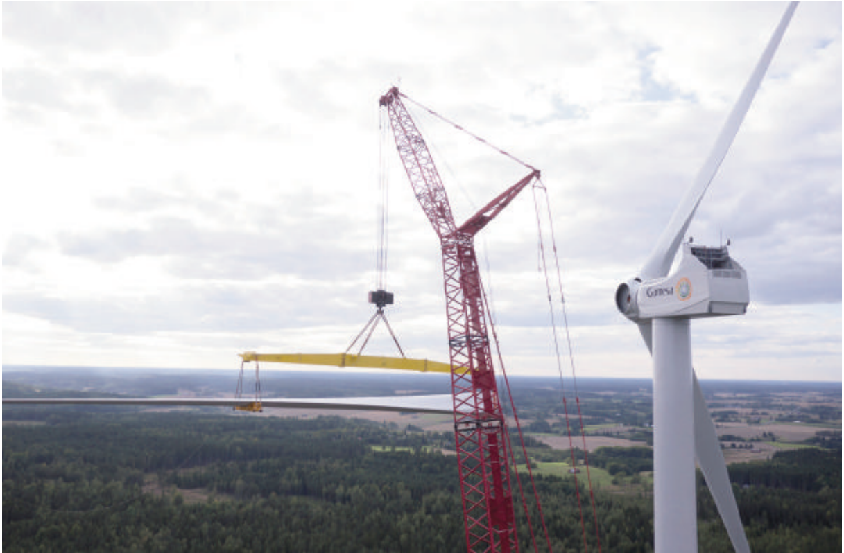
Assembly of the first Gamesa wind farm equipped with 5-MW turbines (Salo, Finland).
