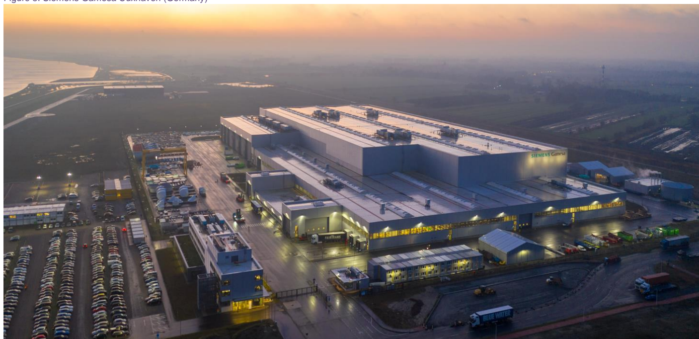
Figure 5. Siemens Gamesa Cuxhaven (Germany)
